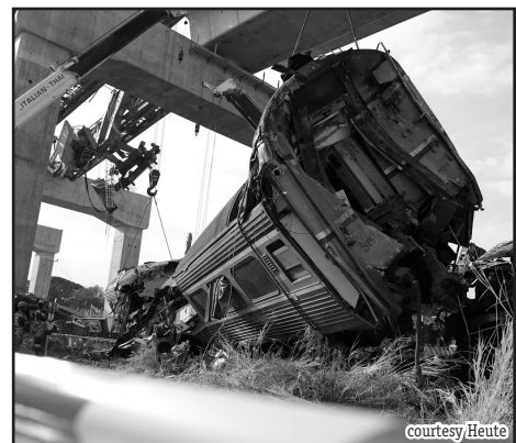
COLLAPSE: A train in Thailand crashes following crane fall.
