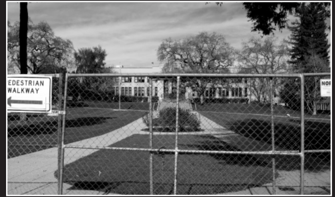
SOD TAKES HOLD: The most time-consuming part of the process from here on out is the sod.
